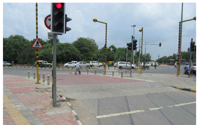
Slowing of vehicle speed through traffic calming measure like raised table top crossing. Location: Delhi Source : www.itdp.com
