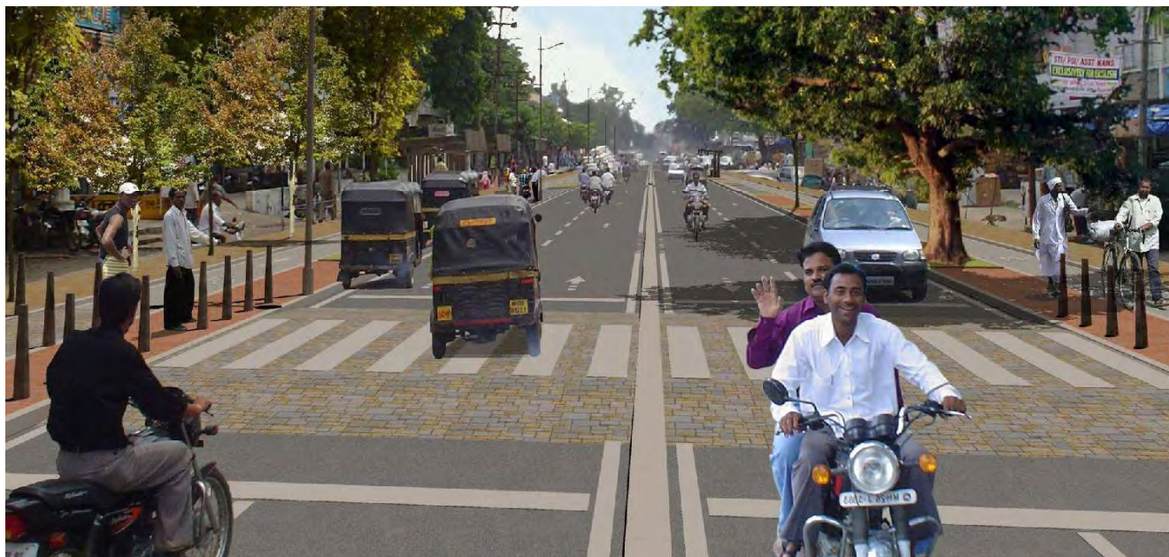
Insertion of table top crossing , facilitating slow down of motorised vehicles and safe crossing with universal accessibility. Delhi BRT ; Source :TRIPP
