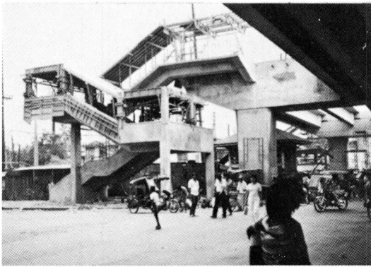
Fig.3 駅の階段 Stairs of LRT station
