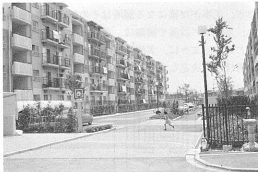
Fig. 2 出入口のハンプ Humps at the entrance and exit
