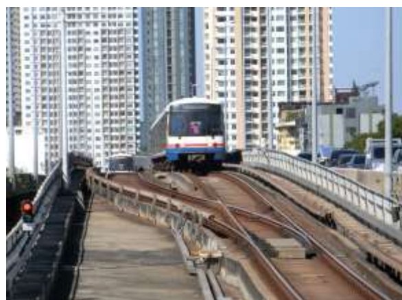
高架通勤鉄道 Elevated Railways (BTS, Bangkok)
