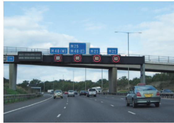
Figure 6. Example of lane-based variable speed limits (U.K.)
