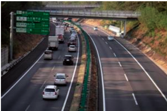
Figure 7. Increase to three lanes between the Otowa-Gamagori Interchange and the Toyota Junction on the Tomei Expressway (source: NEXCO Central Nippon Expressway Co., Ltd. press release)
