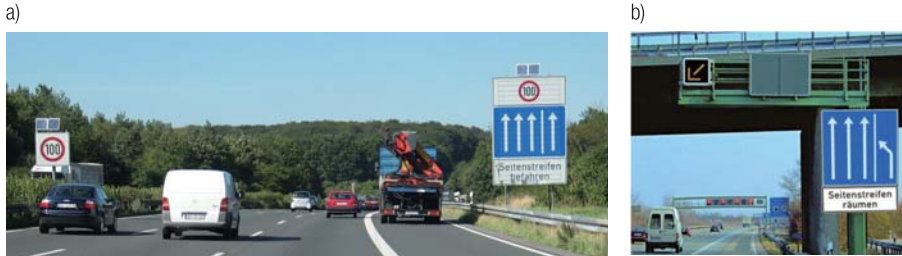
Figure 15 a) Hard shoulder running (HSR) b) End of HSR section
